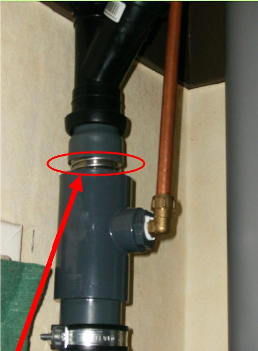
Section showing part of the ribbed heat exchange area between the hot waste water running down and the cold supply water.
