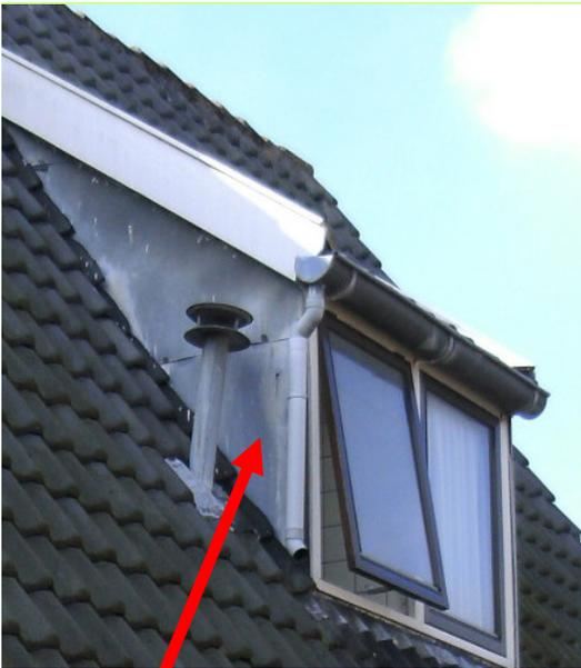
Health hazard: Exhaust vent for flue gas from kitchen gasburner directly beside dormer window.
